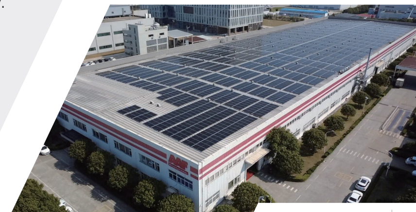
Solar Panels at AAF Suzhou Factory
