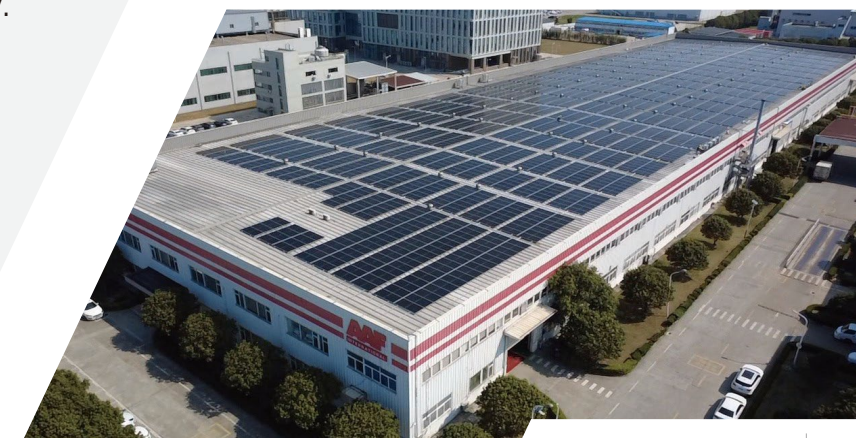
Solar Panels at AAF Suzhou Factory
