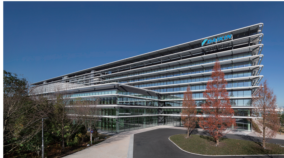
Daikin Technology and Innovation Center (TIC)
