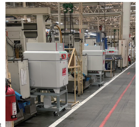
Oil Hunter™ at customer's plant
