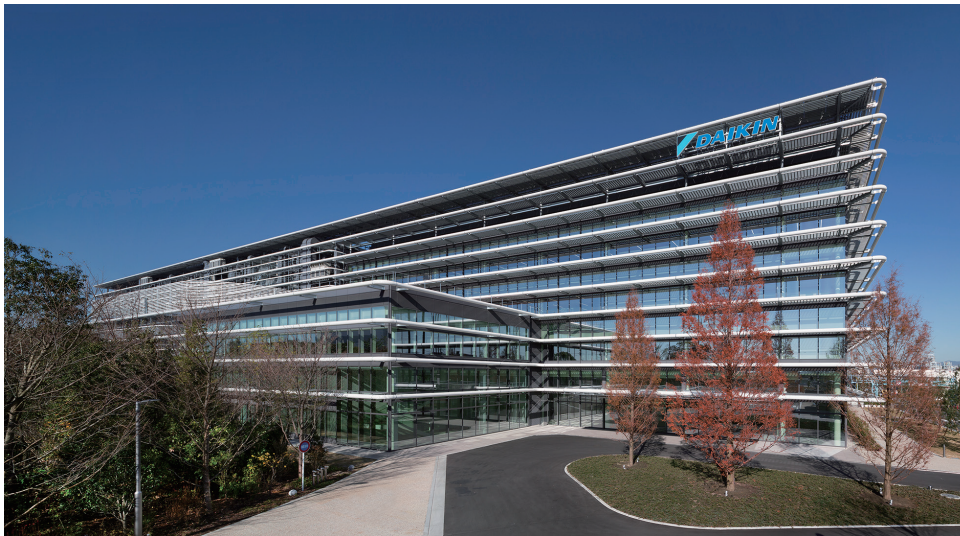
Daikin Technology and Innovation Center (TIC)
